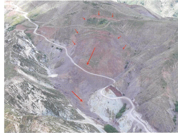
⑥ Landslide in Yesilyayla with long travel distance
