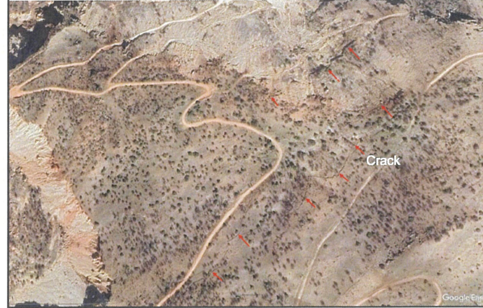
A close view of the cracks
