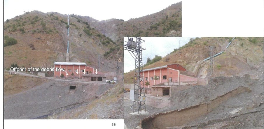
⑥ Landslide in the area near Mutlu village: multiple disasters
